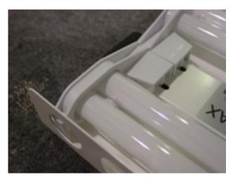
Slide the plastic end cap over the end of the fluorescent tube.
