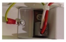
Using a straight blade 2.5 mm (flathead 3/32") screwdriver, depress the grey wire retainers and withdraw the RED (live), white (neutral) and green/yellow (earth/ground) wires on the left side of the ballast. Next, remove the M4 nut and washers holding the ground wire in place, and set aside.
